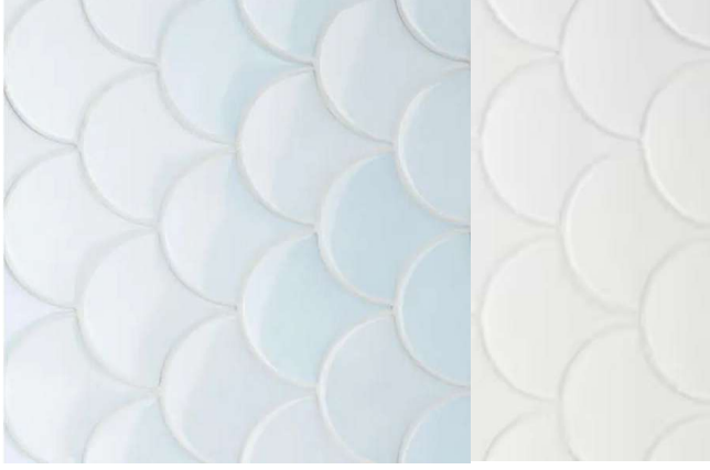
SHOWER WALLS Scallop shaped tile TOP 6' Blue BOTTOM 4' WHITE (transition with the rounded tile edge not cut edge)
