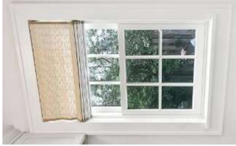
CASED WINDOW STYLE 4" Flat casing with raised edge detail, Sill ear to extend into casing, but not beyond
