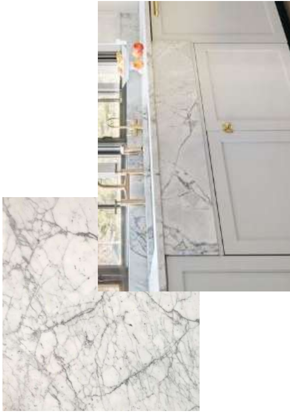
MITERED APRON FRONT At sink (continue edge detail across front like image)
