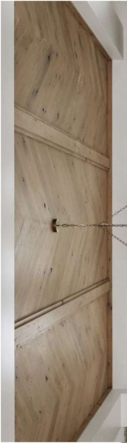
CEILING TREATMENT Herringbone Stained Clear Pine with trim, EXECUTE EXACTLY LIKE IMAGE
