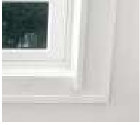
CASED WINDOW STYLE 4" Flat casing with raised edge detail, Sill ear to extend into casing, but not beyond
