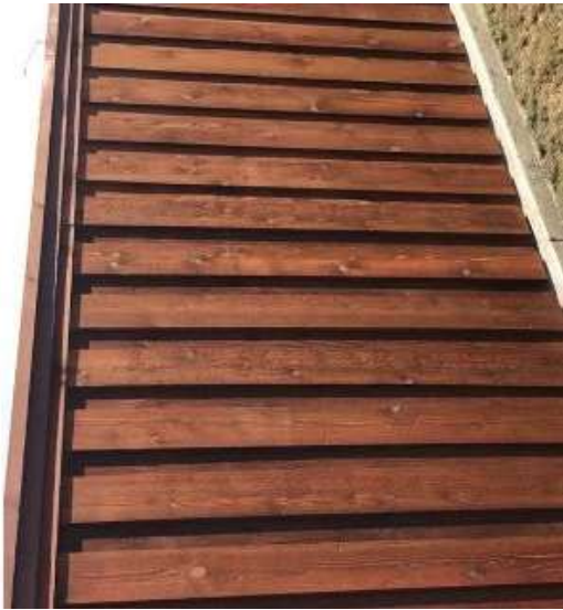
FENCE DETAILS VERTICAL BOARD ON BOARD
